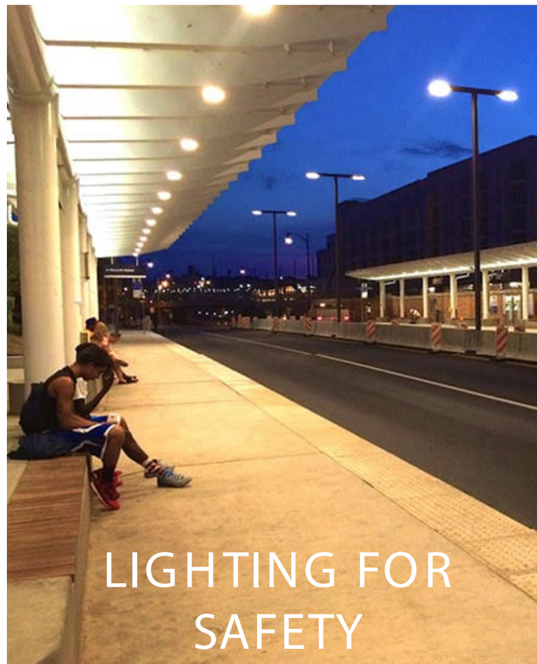
Station Lighting from E. Liberty
